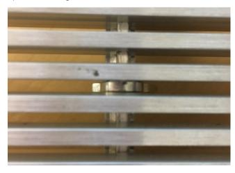
STEP 2: Slide core clip removal tool (CCRT) between the core bars of the grille where the first clip is located. Slide CCRT against core clip and pull up so the bottom of the CCRT opening is against the core clip.
